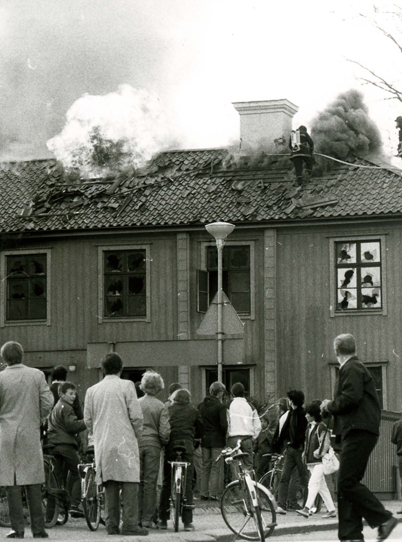
The fire at the Foundation Secretariat in 1982.
